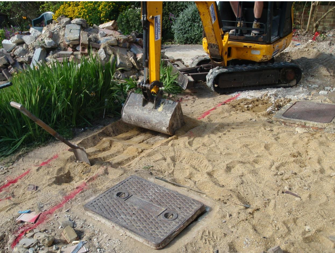
Plate 4. Foundation trench (looking SW)
