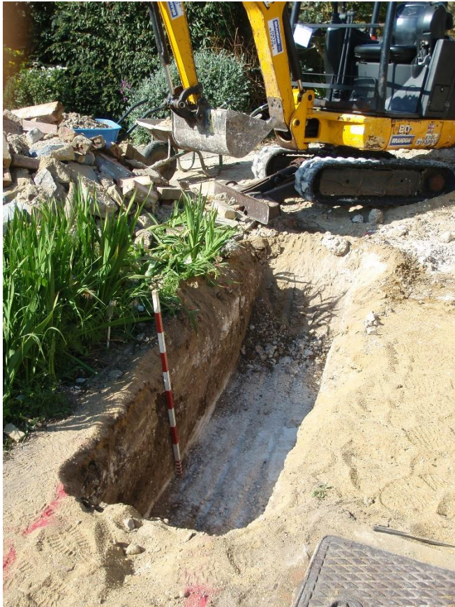
Plate 5. Foundation trench (looking SW)
