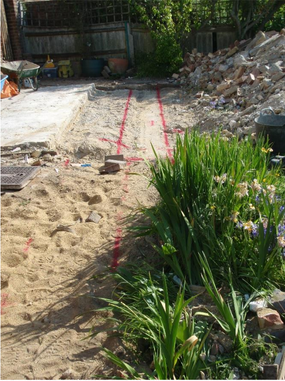
Plate 3. View of foundation trench (looking east)
